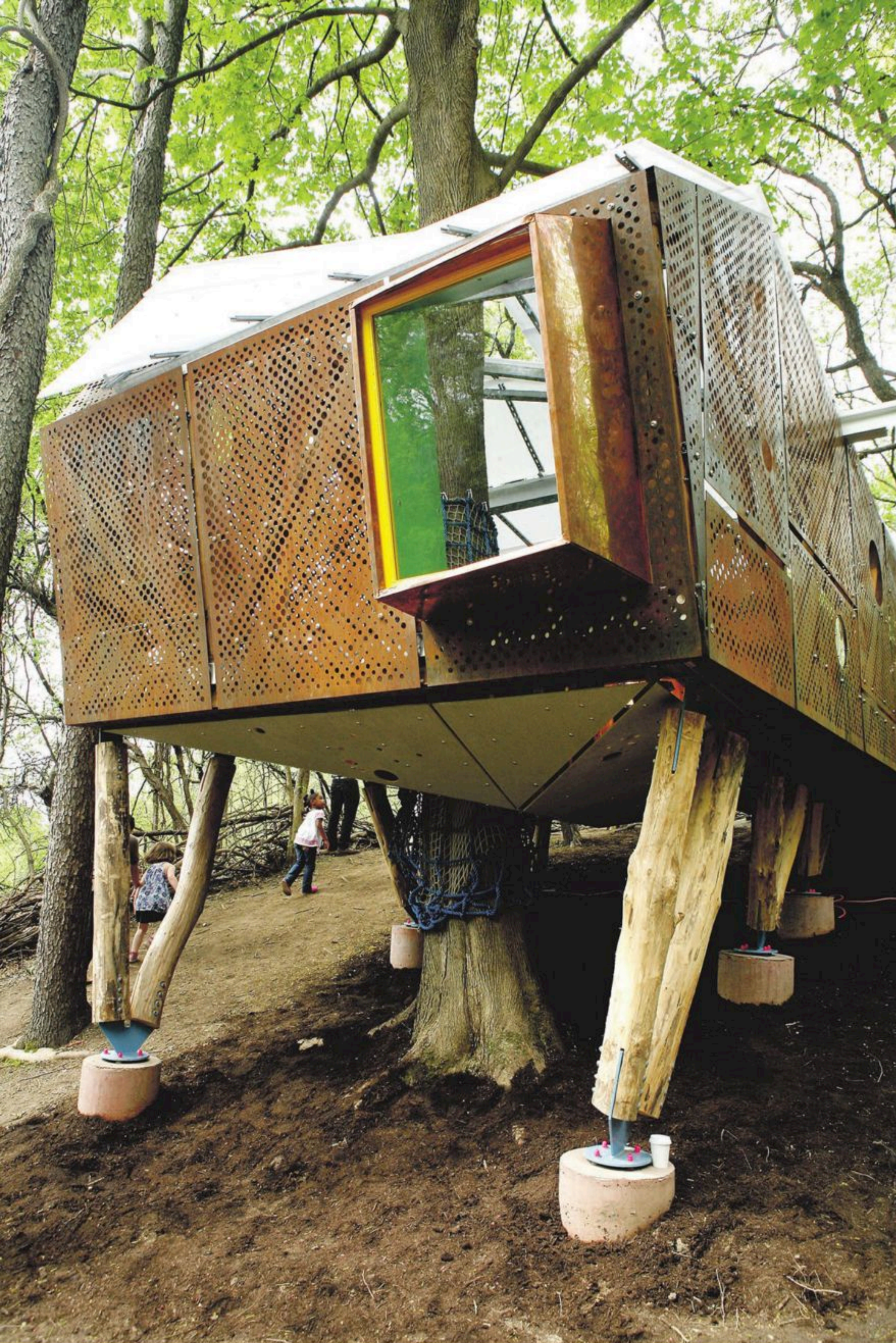
Ready for play: The Play Perch is a trapezoidal structure shuttered in steel panels and topped with plexiglass. The outdoor learning space includes a small auditorium space and a wheelchair-accessible ramp. Below, a youngster helps build it.
